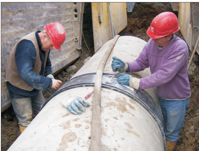
Installation of MÜCHER TITAN XL Couplings: quick & easy
