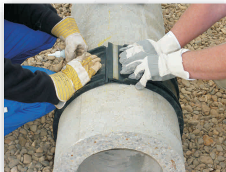
C. Press on top part of sleeve for approx. 10 seconds
