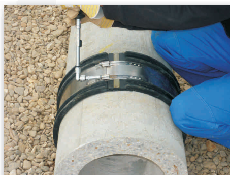
E. Assemble shear band and tighten clamps to recommended torque, see product label
