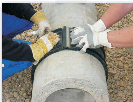
C. Press on top part of sleeve for approx. 10 seconds
