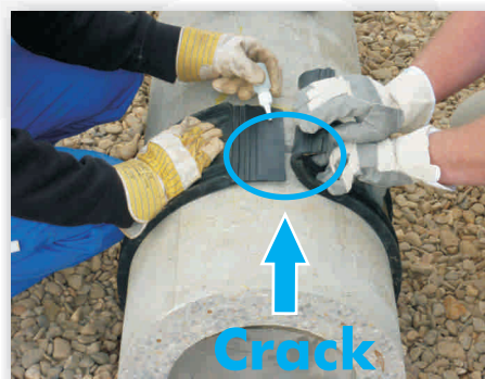
B. Protection goggles and gloves should be worn - coat rubber glue to the bottom of the sleeve
