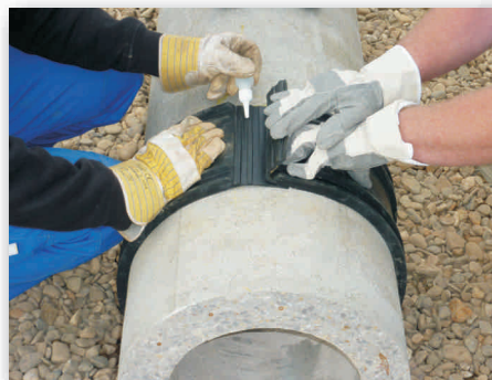
D. Coat rubber glue to remaining free part of sleeve and press on sleeve for approx. 10 seconds
