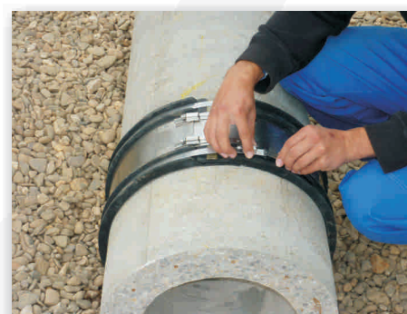
F. Assemble end clamps and tighten the recommended torque, see product label
